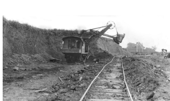
Dam Construction Deer Flat Reservoir
