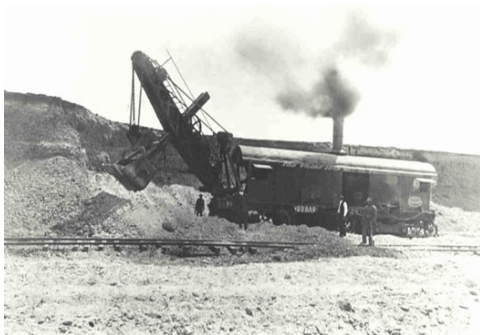
Steam Shovel at Dam 1906
