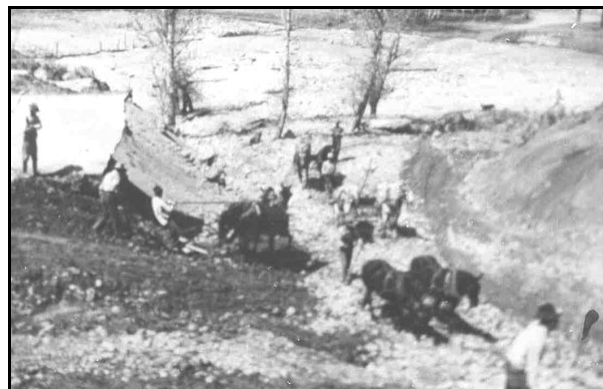
Construction of Phyllis Canal 1915
