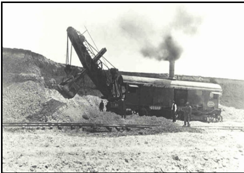
Steam Shovel at Dam 1906
