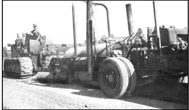
Paving in Nampa Area
