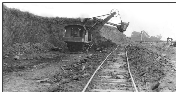
Dam Construction Deer Flat Reservoir
