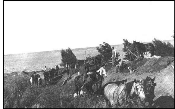
Construction of New York Canal
